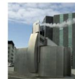
GEOTHERMAL WELL for absorption chillers and desiccant system
